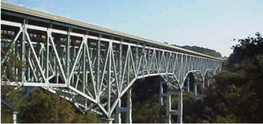
A railway bridge.
